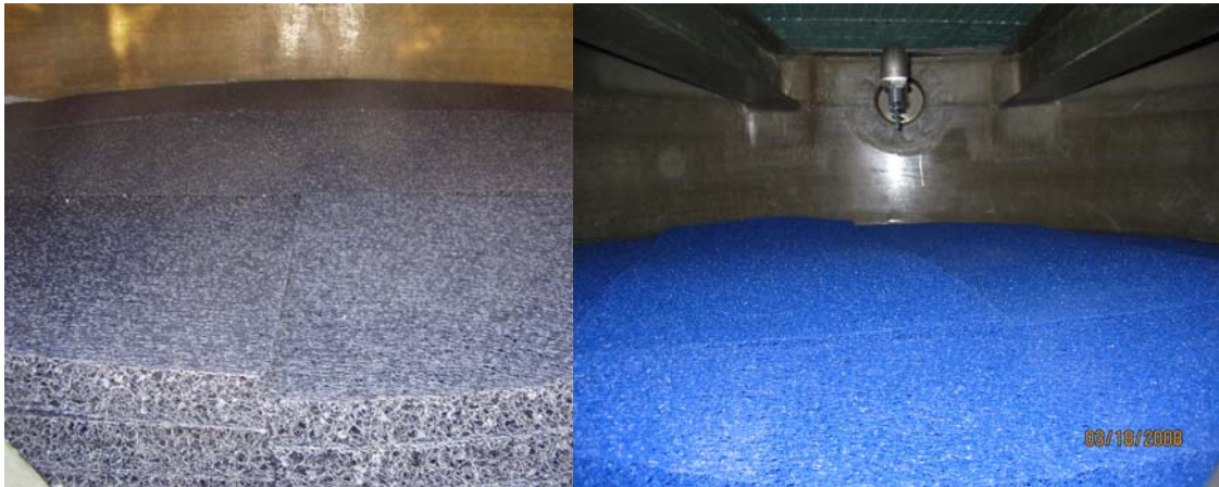
Figure 2. Upper and Lower Media Inside the Vessel
